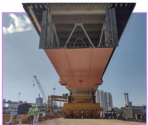
Members in India, Express Global Logistics (EXG) have successfully transported the first of 30 OSDs (Orthotropic Steel Decks) for the Mumbai Trans Harbour Link Project. The deck weighs an incredible 1,362mt and this is the first of 30 that EXG will handle for the project, totalling 40,860mt.
